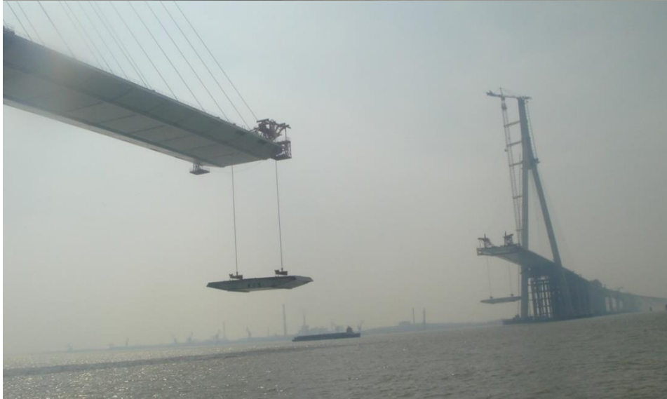
Sutong bridge deck erection gantries, China
