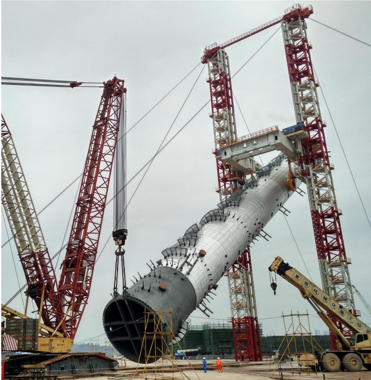
DL-TS3600 jacking tower system, China
