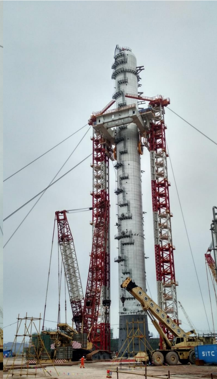
DL-TS3600 jacking tower system, China
