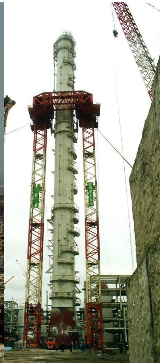
1600 tonne capacity modular jacking tower system, Taiwan
