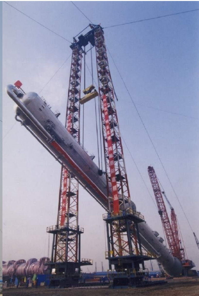
2500 tonne capacity modular jacking tower system, China
