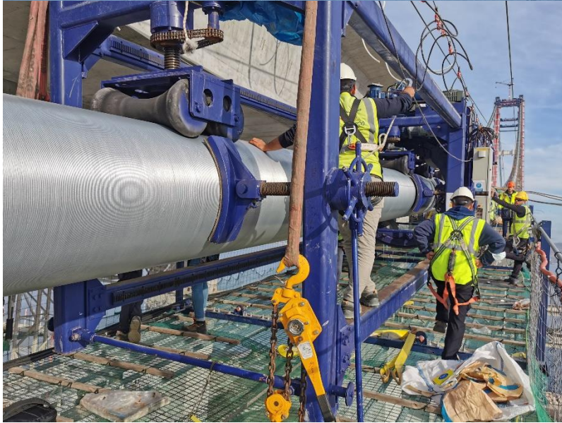
1915 Çanakkale Suspension Bridge, Turkey Main Cable Wrapping Machines
