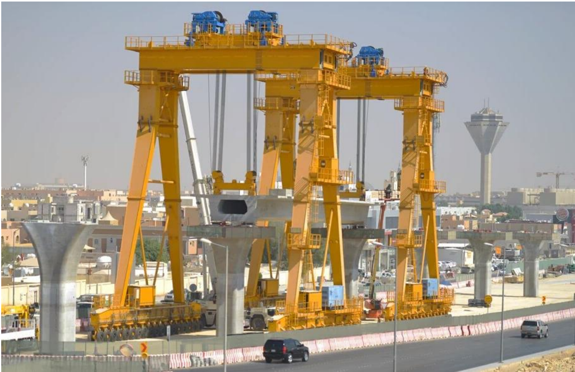
2 x 260 tonne capacity straddle carriers, Riyadh Metro, KSA
