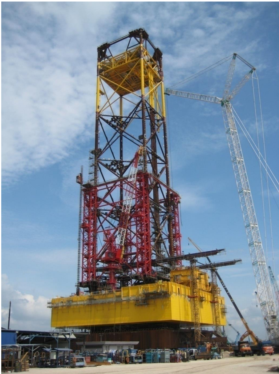
MAARI jacket incremental lifting, Malaysia
