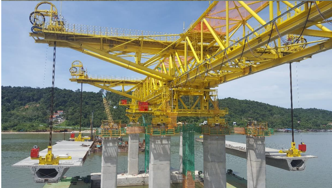
2 x 870 tonne capacity gantry for Temburong Bridge, Brunei
