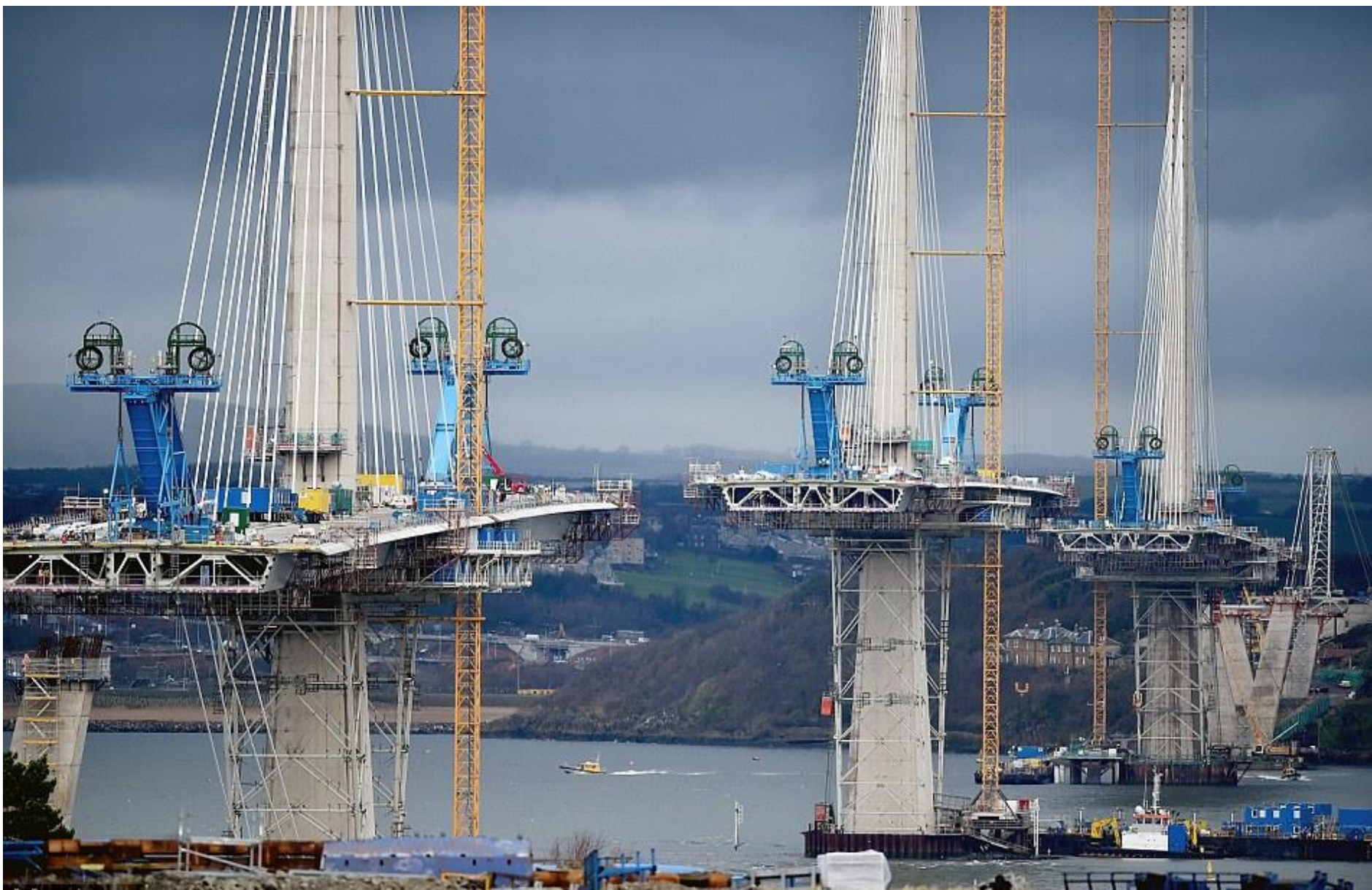
Forth cable stayed bridge deck gantries, UK
