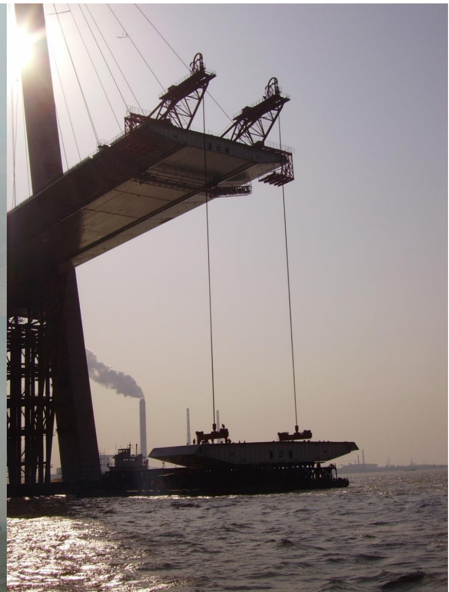
Sutong bridge deck erection gantries, China
