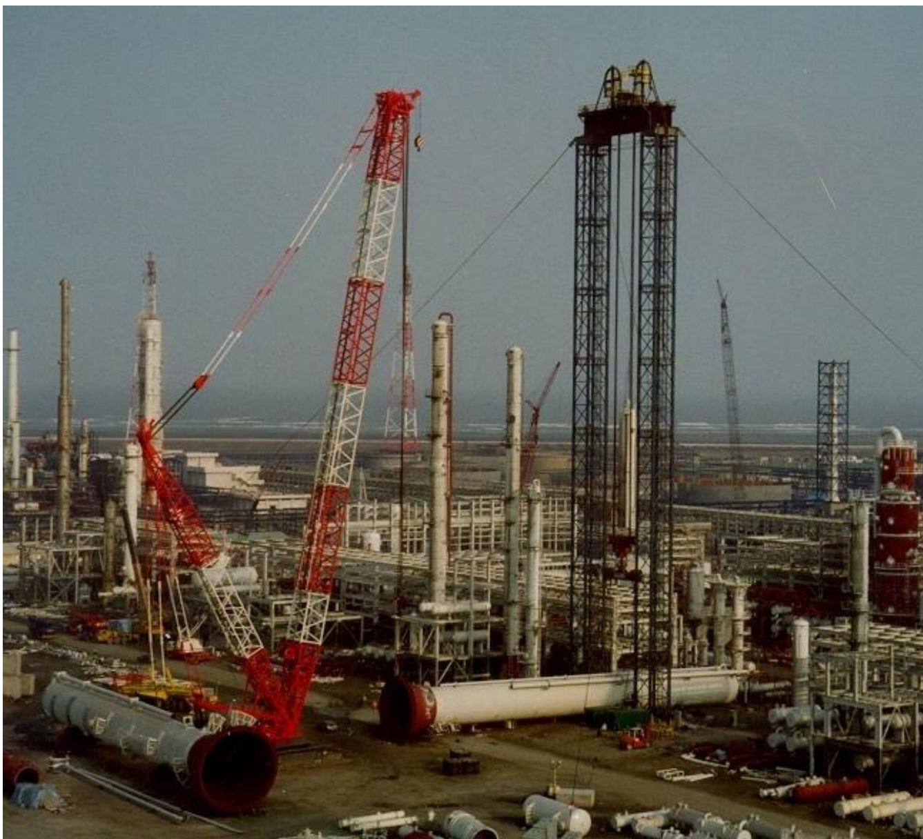
1600 tonne capacity modular jacking tower system, Taiwan
