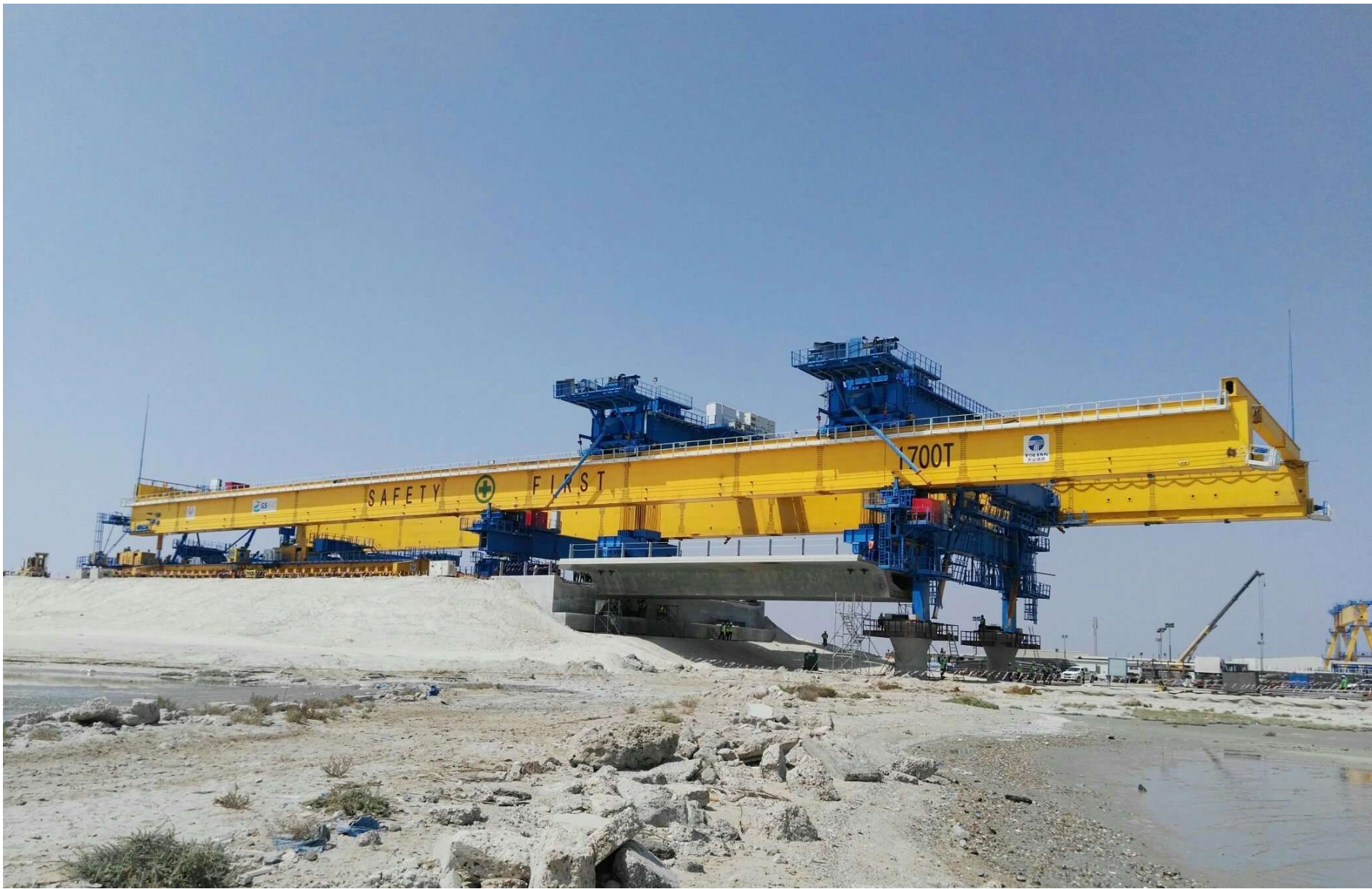
Doha Link gantry, 60m 1700 tonne capacity, Kuwait
