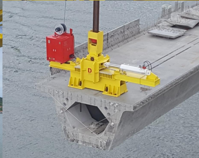
2 x 870 tonne capacity gantry for Temburong Bridge, Brunei
