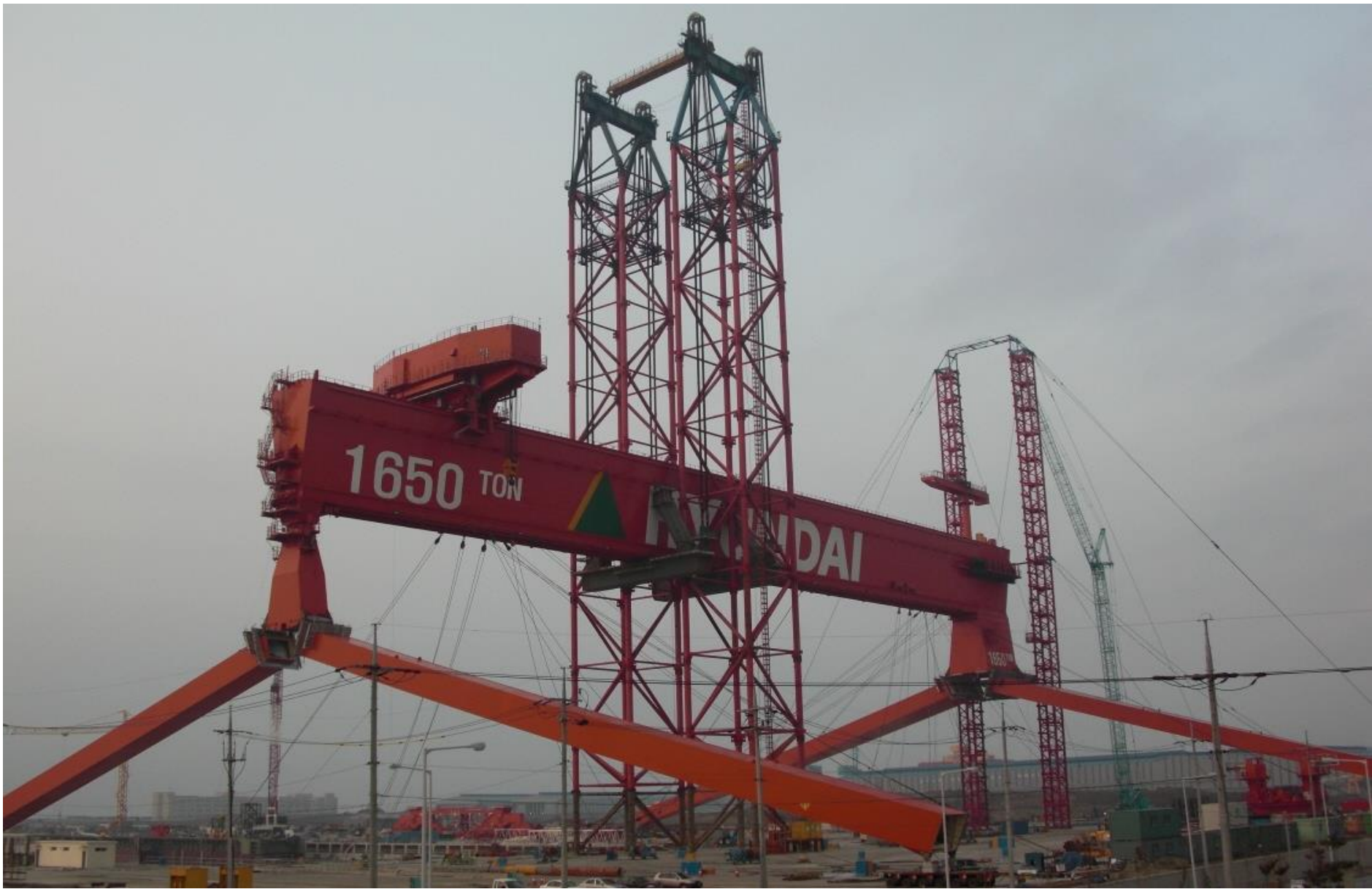
Goliath crane erection, Gunsan, Korea
