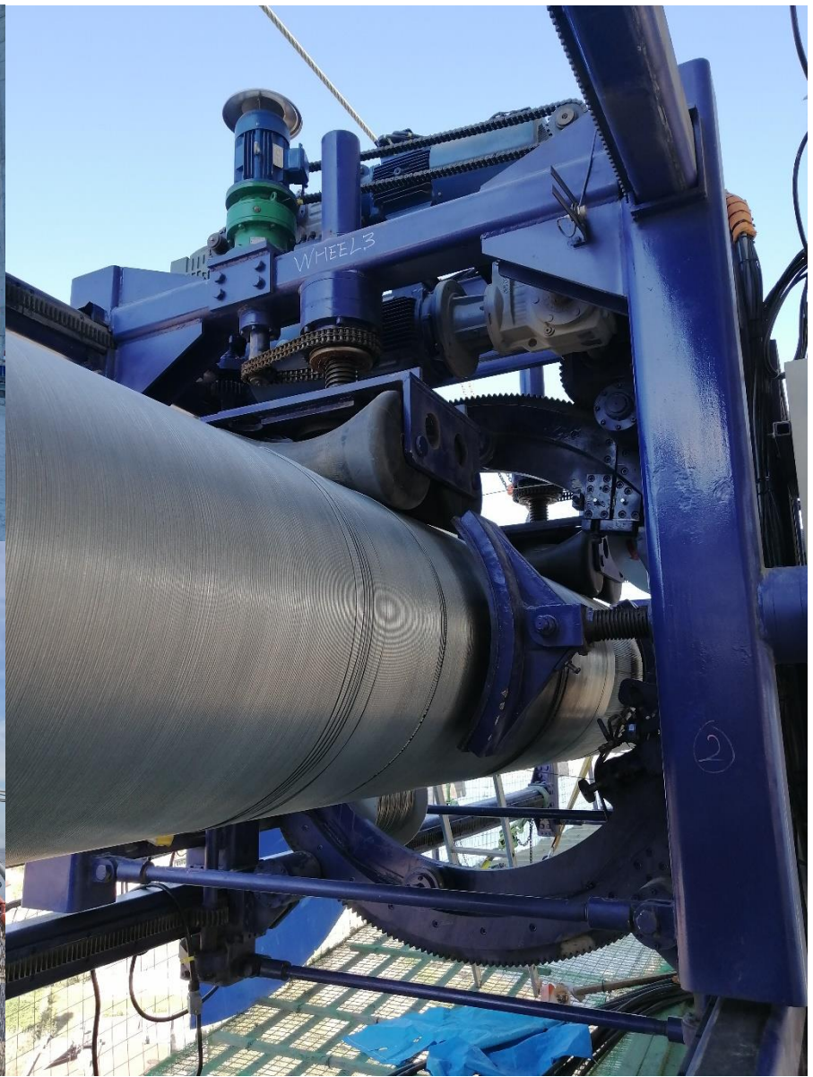
1915 Çanakkale Suspension Bridge, Turkey Main Cable Wrapping Machines
