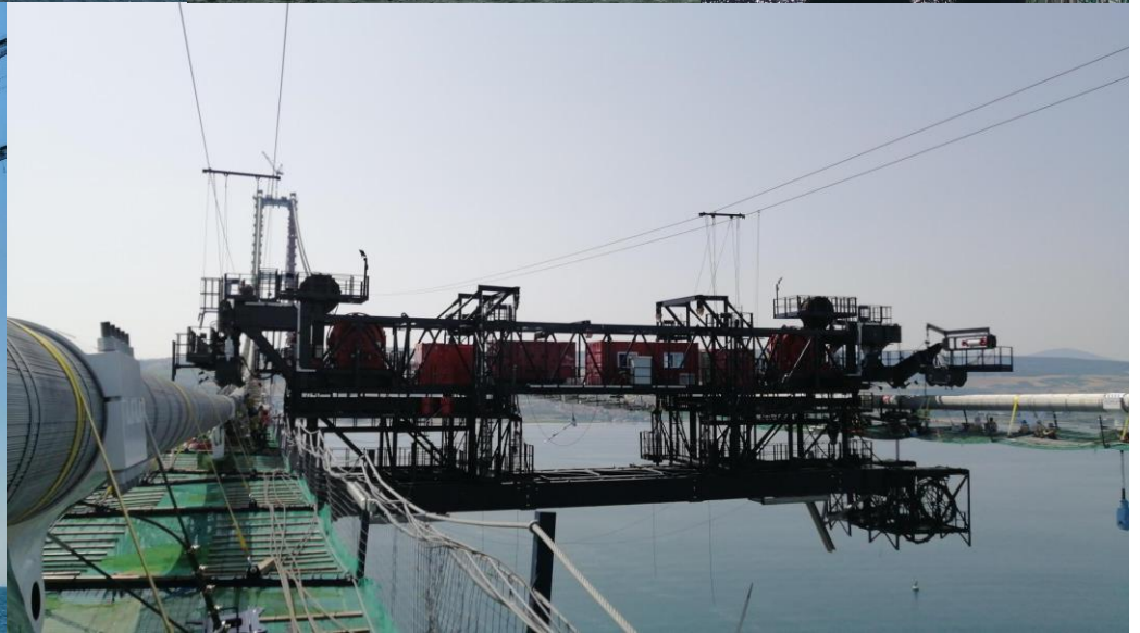
1915 Çanakkale Suspension Bridge, Turkey Deck Erection Gantries
