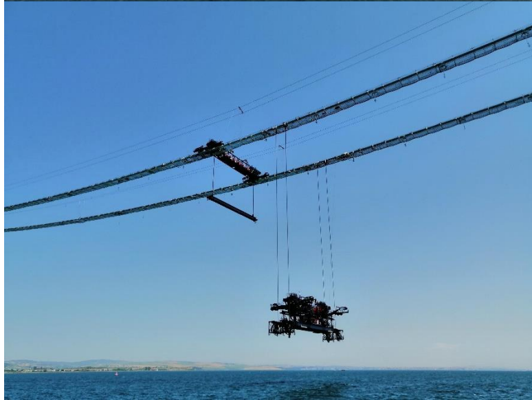
1915 Çanakkale Suspension Bridge, Turkey Deck Erection Gantries
