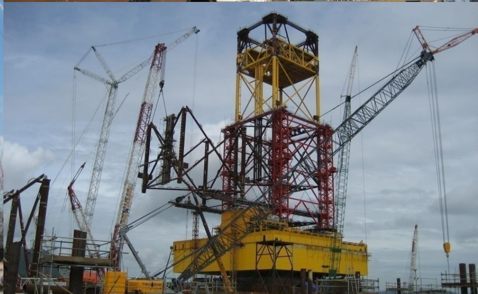
MAARI jacket incremental lifting, Malaysia
