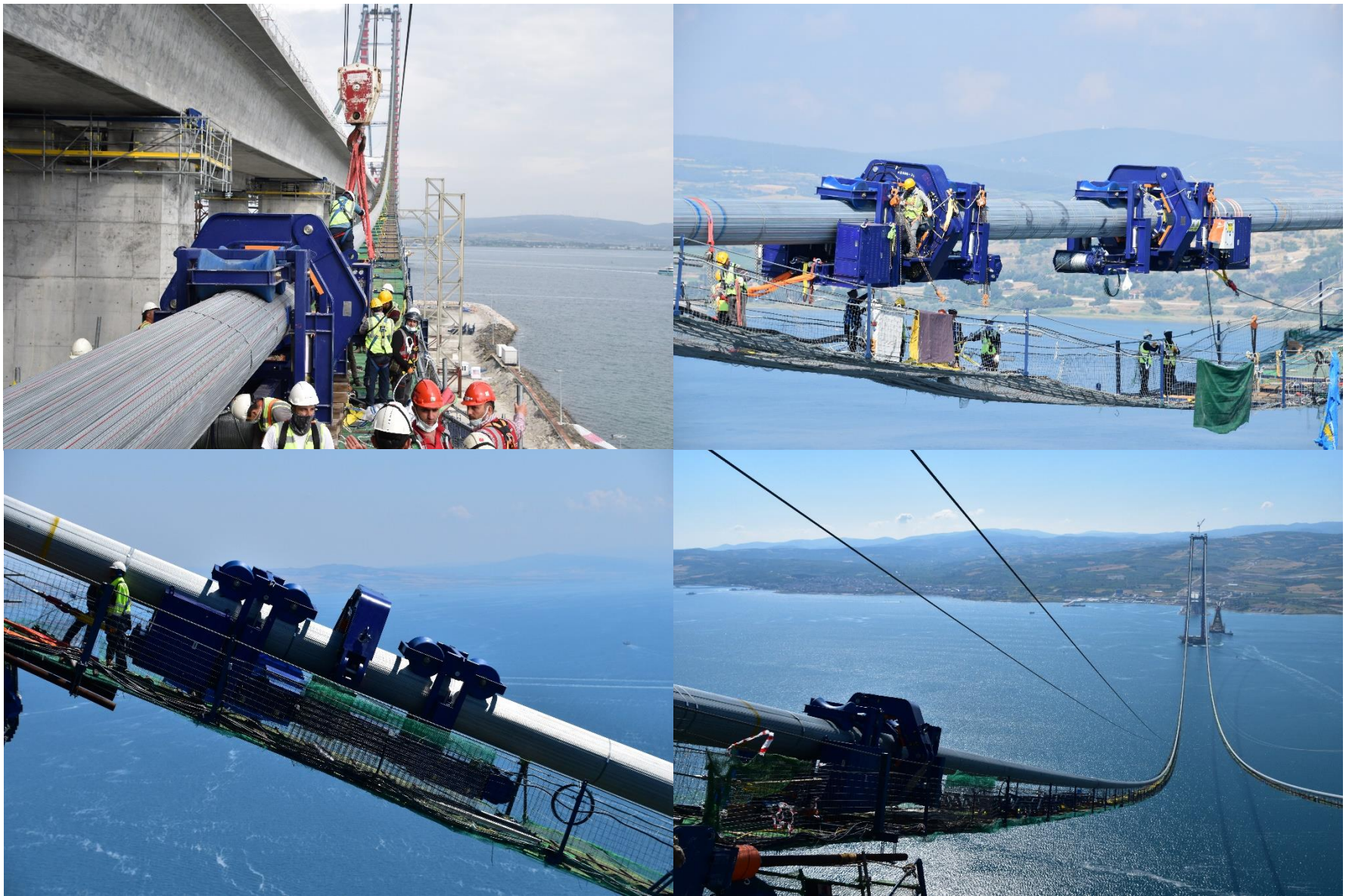
1915 Çanakkale Suspension Bridge, Turkey Main Cable Compaction Machines
