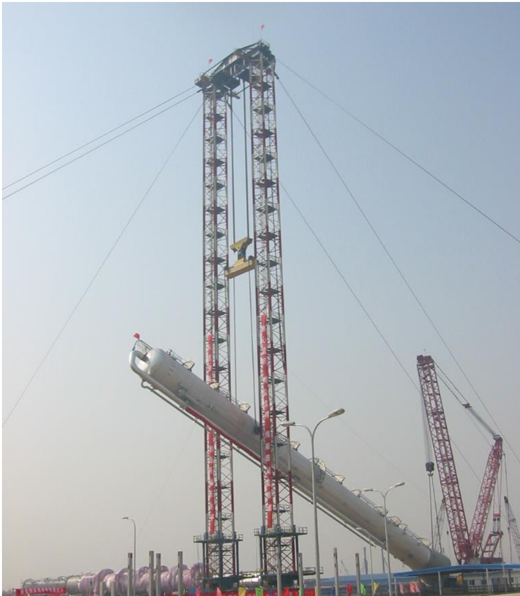
2500 tonne capacity modular jacking tower system, China
